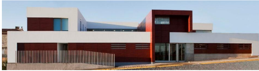
Img. 31 Fachada principal
