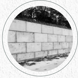
F352 . Muro Block
