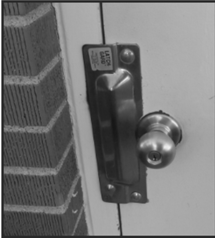
Figure 11 Latch Guard Installation (Photo by Ernie Hayden)
