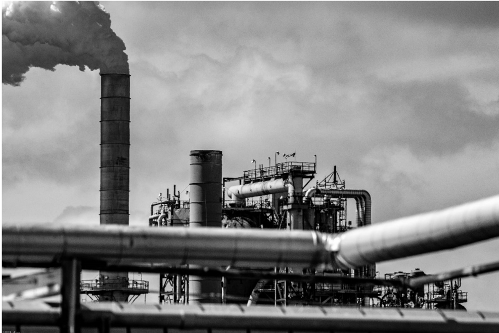
Figure 5 Example of Seismic Pipe Hangers (Photo by Ernie Hayden))
